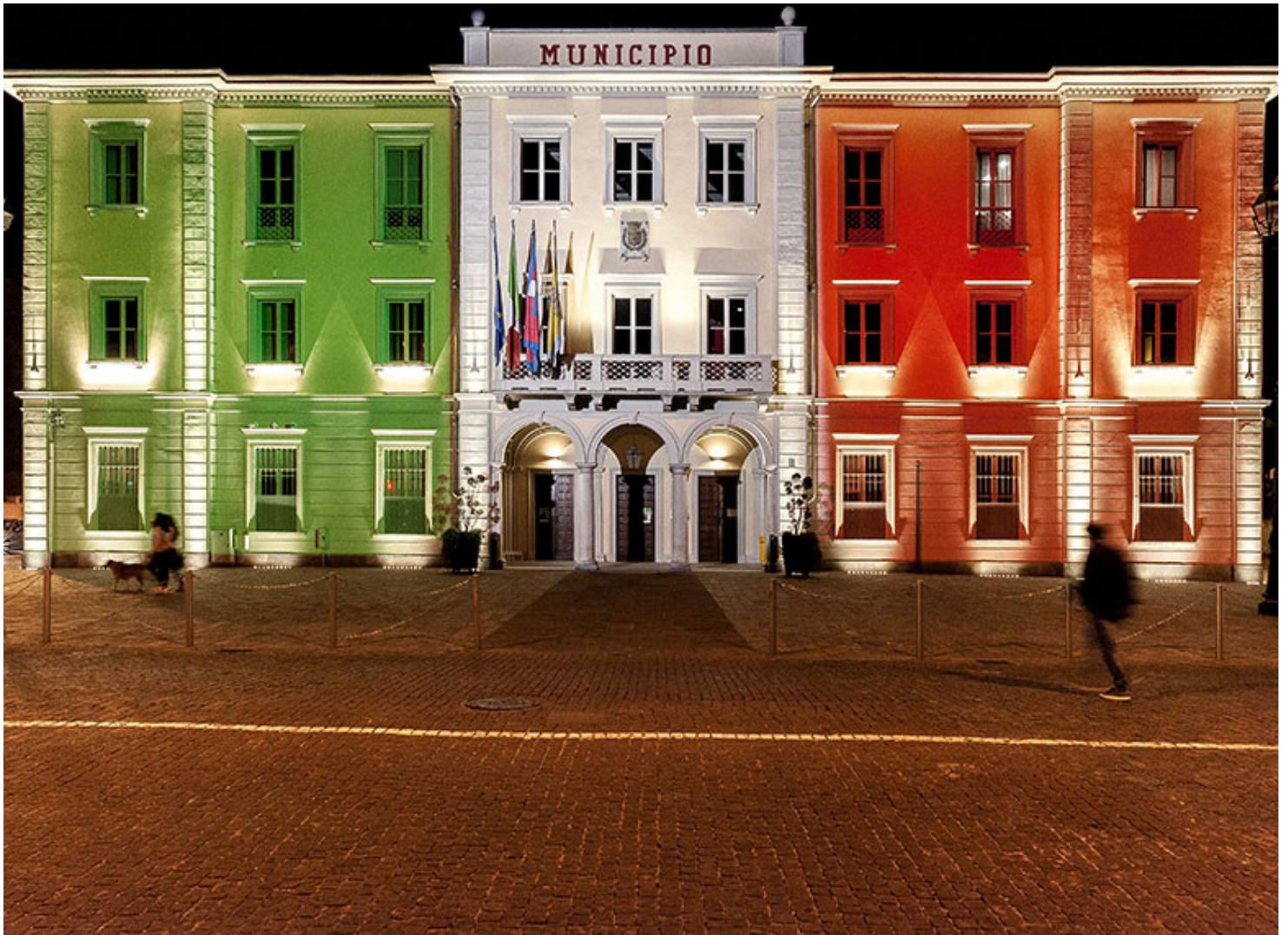
Architectural Outdoor - Town Hall of Nichelino, Turin, Italy
